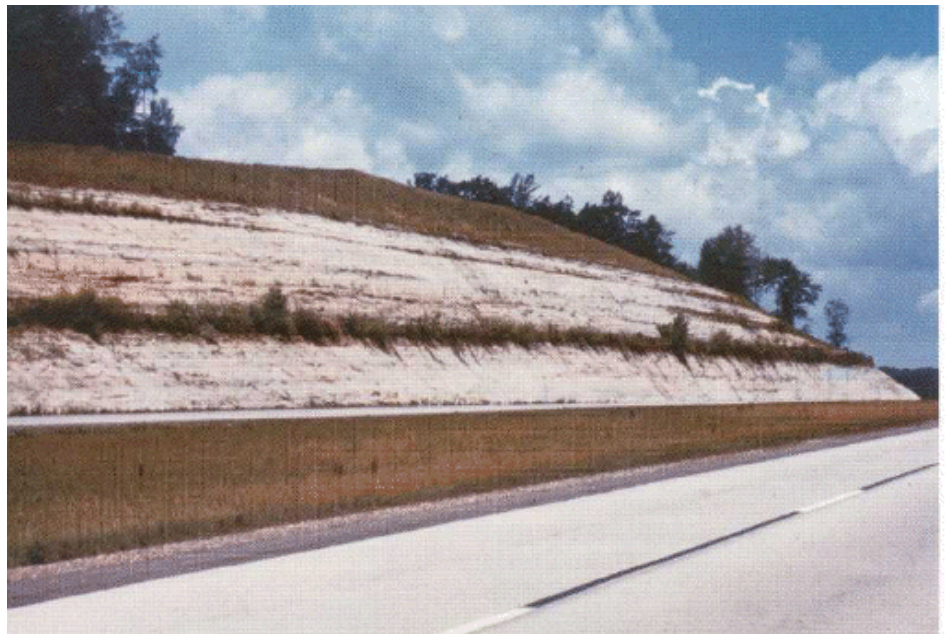
Figure 3. Road cut showing a horizontal plain of groundwater discharge (Modified from Waller, 1988).
